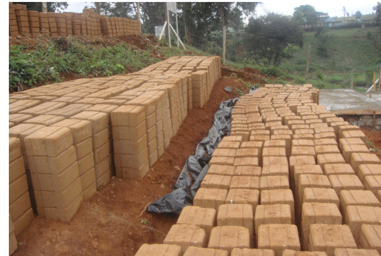
Interlocking Stabilized Soil Blocks
