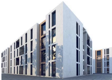
Apartment buildings, Rwanda
